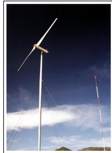
***Exhibit 4.5-3 Two-Bladed Downwind Wind Turbine***
