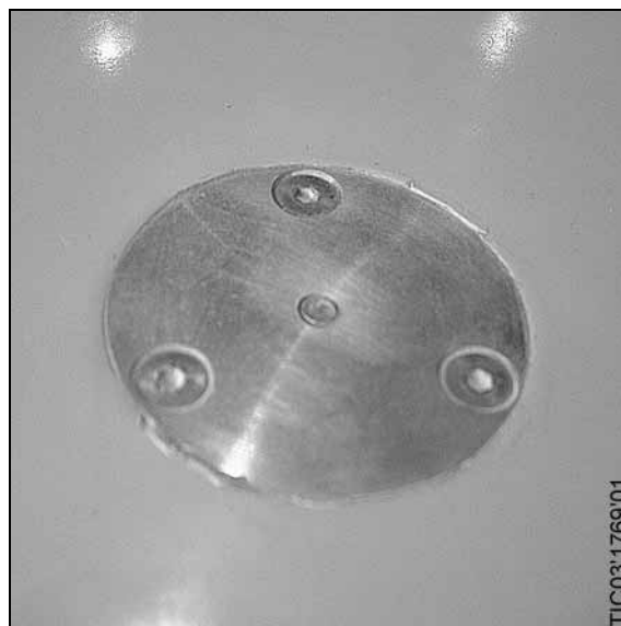
Close-up picture of lightning receptor on blade
